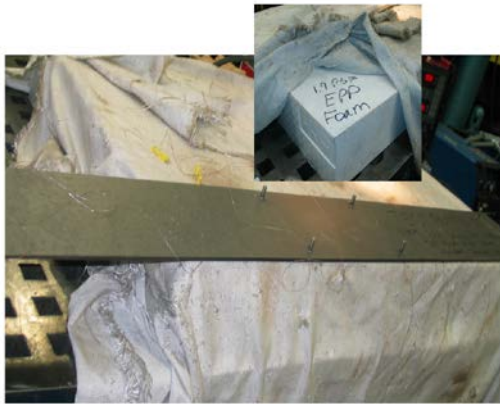
Figure 15: Stud Welding Setup with View of Foam Under Weld Blanket
