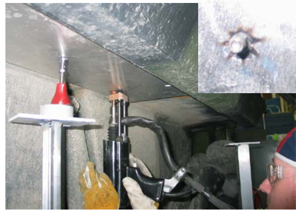
Figure 17: Stud Welding 1/4 stainless steel studs onto the LAV-25A2
